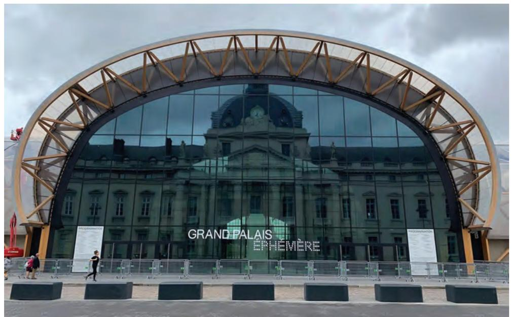
In Mathis company hangars, operations dry wood, cut planks into pieces, and glue them together. The only large machine is a press that bends huge pieces of laminated wood up to 45 meters long into arches for roof supports. The material is so pliable that the wood can gain and retain the desired shape after just a day in the press before being shipped to a construction site.
