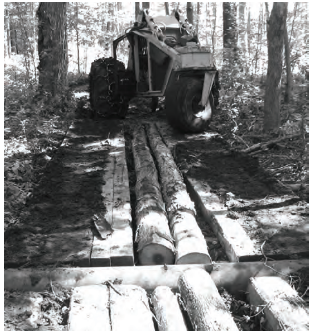
Above: Skid trail before protection. Below: Crane mats laid down to prevent erosion.
